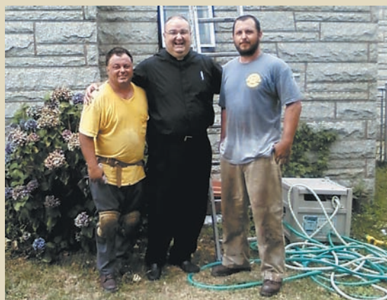
St. Barnabas Pastor Father John Babowitch stands with workman in front of the nearly completed roofing project.
